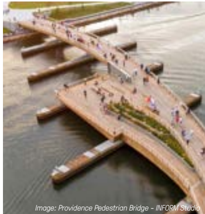
Image: Providence Pedestrian Bridge - INFORM Studio
